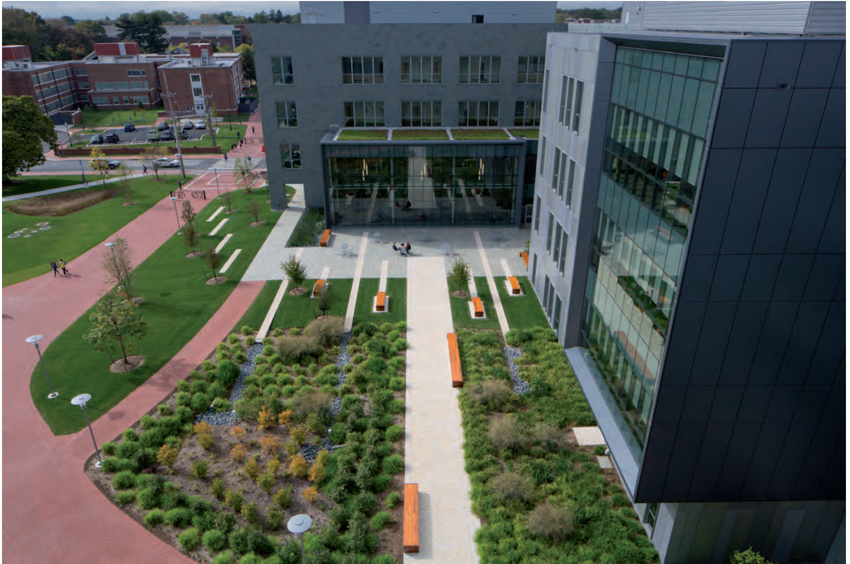
Building sites and open space improvements provide opportunities to visibly express sustainable site features such as stormwater management through green roofs, permeable planters, and bio-retention ponds. (University of Delaware Interdisciplinary Science and Engineering Laboratory and plaza)
